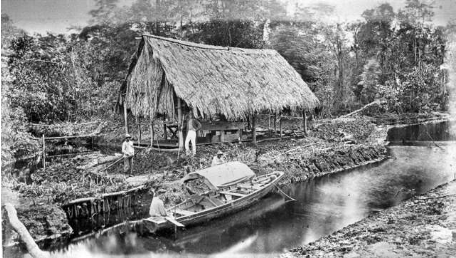
Lamaha Canal under construction
